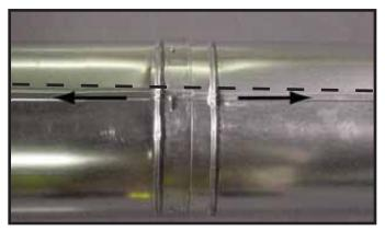
Figure 10.11 Align and Disassemble Vent Sections
